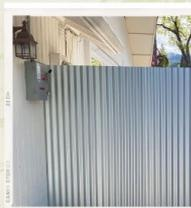
Use noncombustible materials for the portion of the fence that connects to the house to prevent fire spread.
