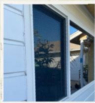
Fit dual-paned windows with at least one tempered glass layer to withstand fire-induced breakage
