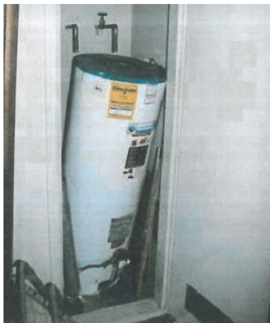
Photo of water heater failure in 1994 Northridge Earthquake. COURTESY OF EXPONENT
