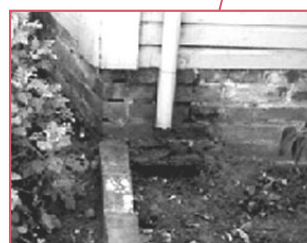
Continuous unreinforced stone or masonry foundation
