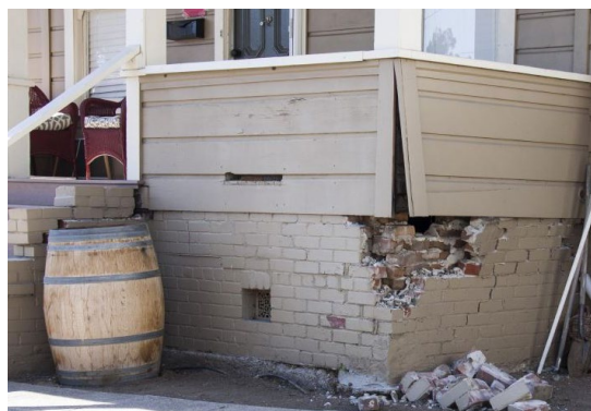
Photo of damage to unreinforced masonry building in South Napa Earthquake.
