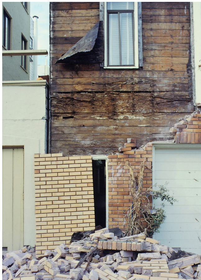
Brick masonry veneer fallen off of home exterior.
