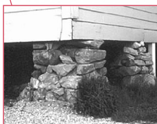
Isolated stone or brick piers
