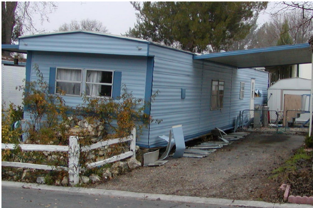
Manufactured home that has fallen off of support piers. PHOTO COURTESY OF KELLY COBEEN
